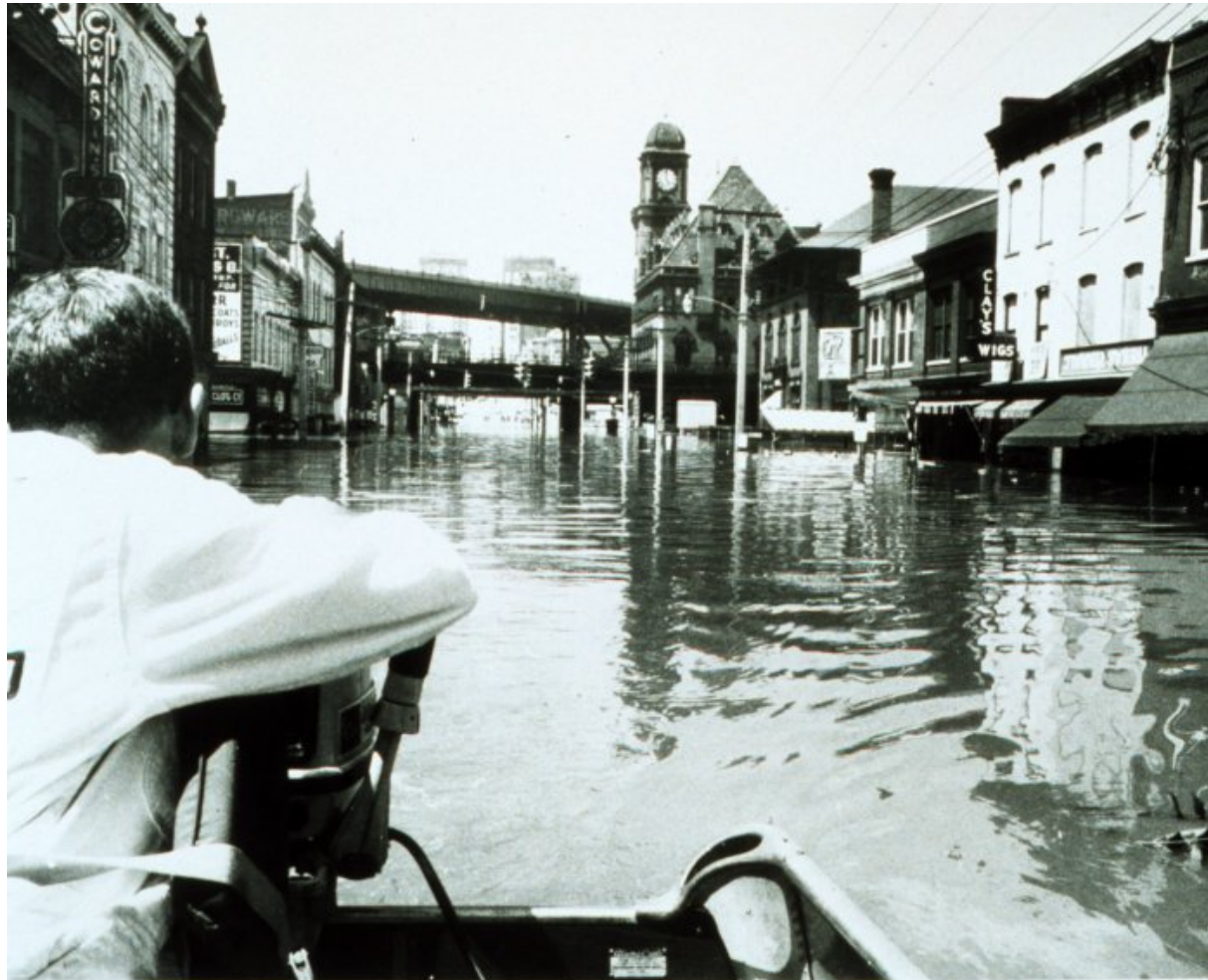
James River at Richmond, Va., Main Street Facing West, August 23, 1969 (Courtesy, Richmond Times Dispatch)
